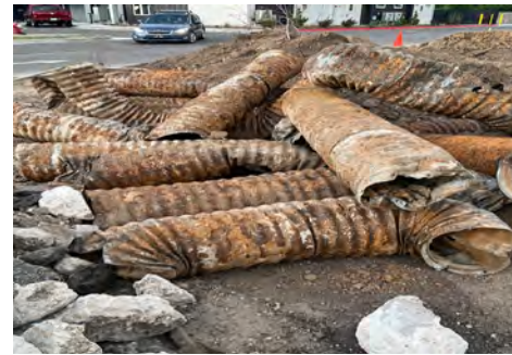
At left and center, crews working to remove the old asphalt and pavement while the weather holds true. At right, crews discovered and removed more than 150 feet of buried culvert pipe that likely dates back to the 1930s. Photos courtesy of Rod Edmonds.
